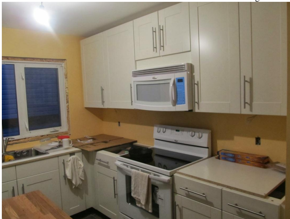
Kitchen almost finished
