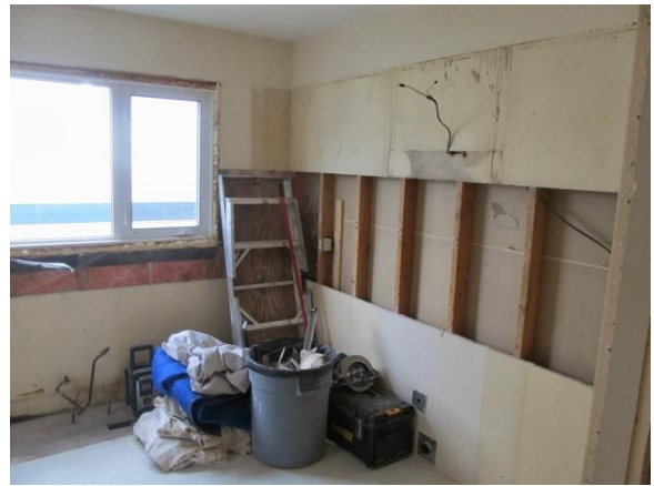
Kitchen during renovations
